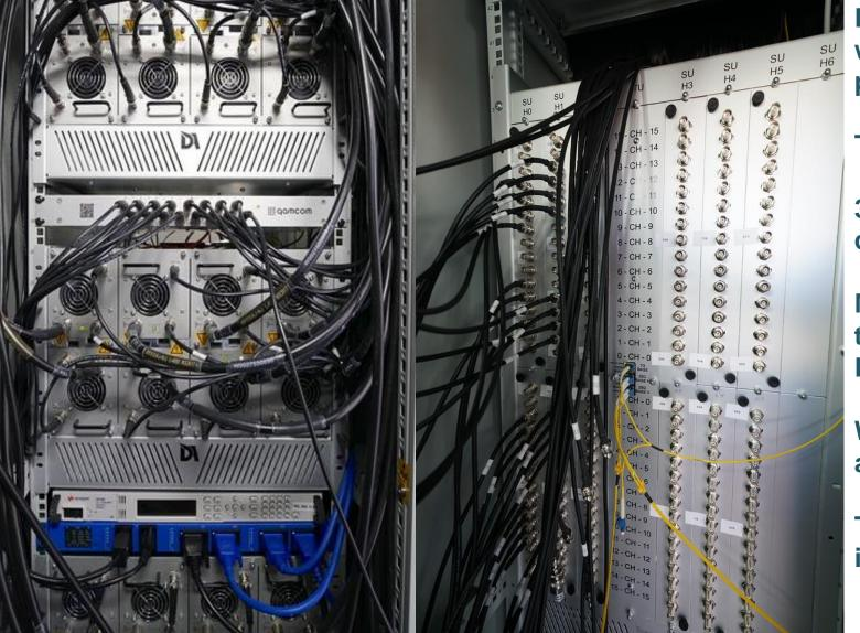
Four Transmit Units (TU) are installed which can drive 16 antennas with two polarizations.
